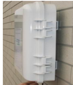
FDB fiber termination box on the wall
